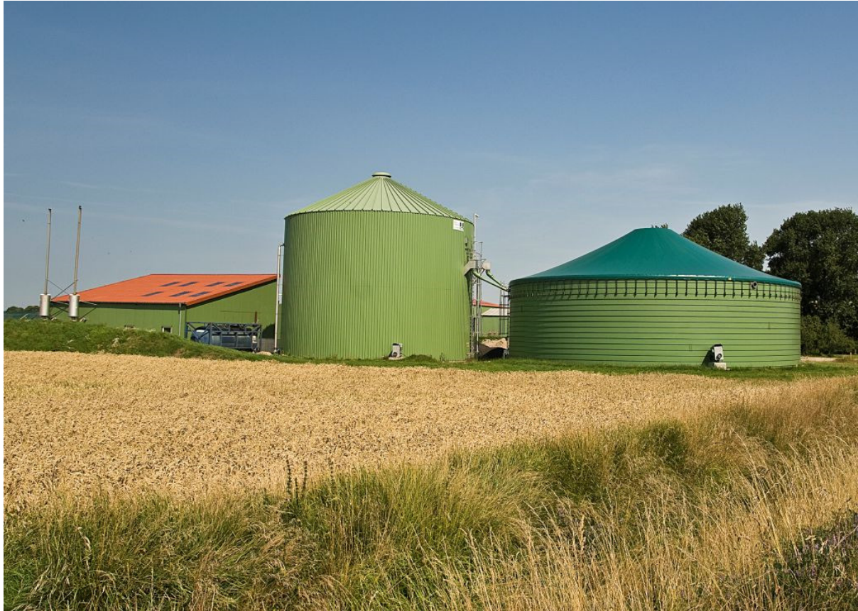
Figure 3: A wet digestion system of approximately 200kWe output
